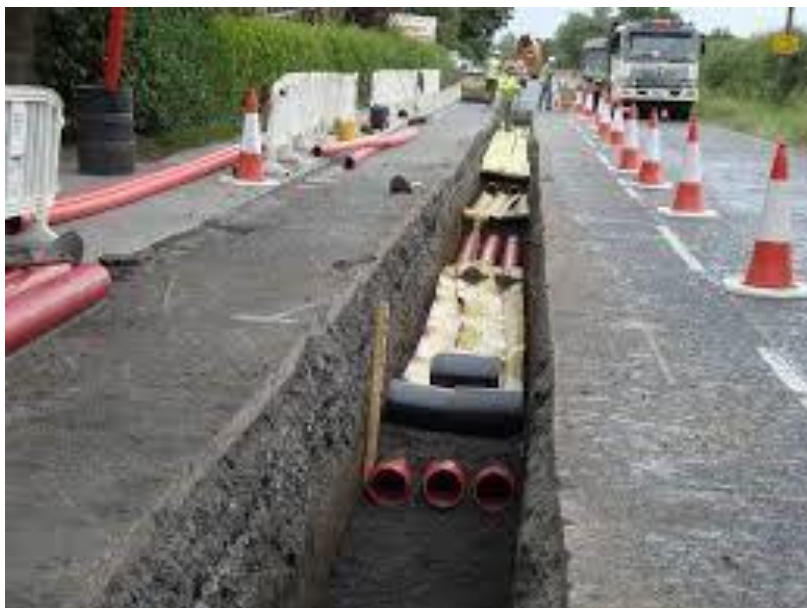
Example of underground cable trench on the Public Road
